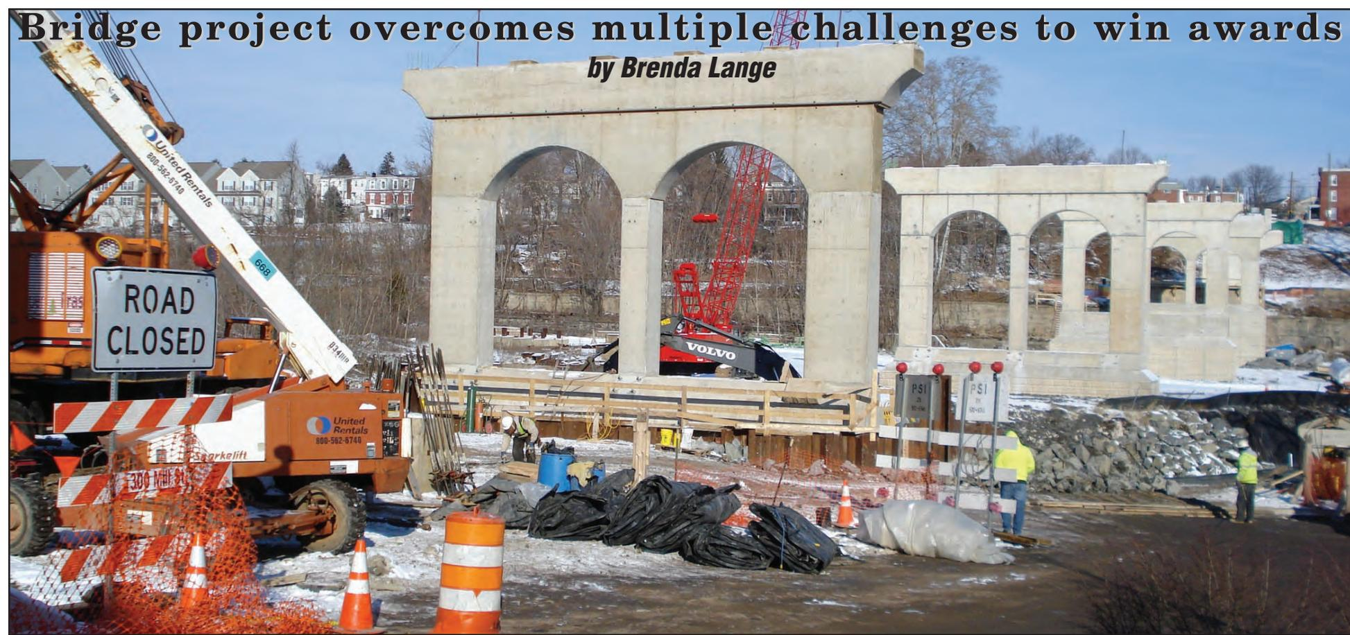
**Concrete piers are in place awaiting the steel decking material.**
